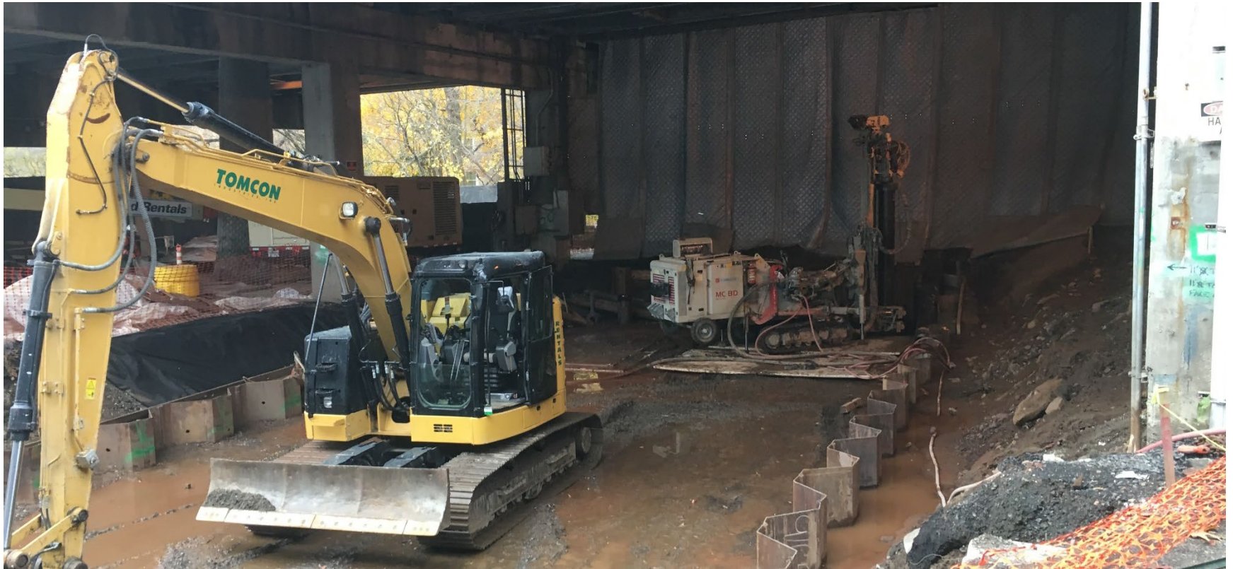
Limited Overhead Room
